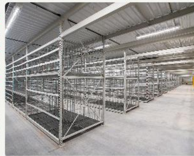
Pick Module Racking
