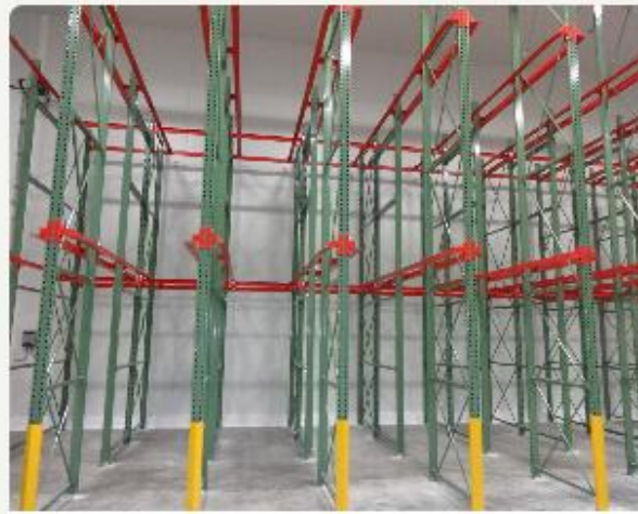
Drive-In & Drive-Through Racking
