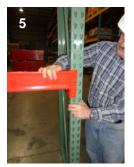
Seat the Beam, as shown in photographs 4 and 5, by engaging the studs in the beam end plate into the keyholes of the column. The beam is correctly seated when the H001 Spring Clip slides into the top of the end plate and can then be locked in place by inserting the stud into the hole in the end plate and column as show in photograph 6.
