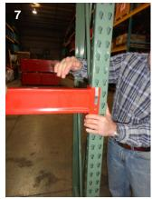
While steadying the Upright Truss with the Beam connected and locked in place, raise another Truss and connect the Beam as previously outlined. and shown as photographs 7 and 8. Continue working in one direction setting up rack bays. Do not set up bays from two ends working toward a center.
