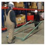
Photographs 1, 2 and 3 show a Truss being raised to its upright position. Make certain the Truss Base does not slide by placing a foot on the Bottom Horizontal brace.
