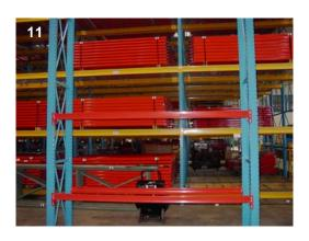
Additional rack bays and beam levels may be added as shown in photograph 11. The rack unit, shown in photograph 12, is now completed and Row Spacers, if desired, may be installed. Row Spacers are used to space rack rows placed back to back. They also act in distributing forces should the rack be struck. Row Spacers should always be installed in line with, or near a Horizontal Truss member.
