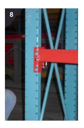
The Beam is correctly seated when the H122 Locking Pin may be inserted, as shown in photographs 7 and 8, through the elongated hole on the Connector.
